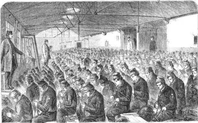
LARGE DAKUM-ROOM (UNDER THE SILENT SYSTEM) AT THE MIDDLESEX HOUSE OF CORRECTION, COLDBATH FIELDS.
